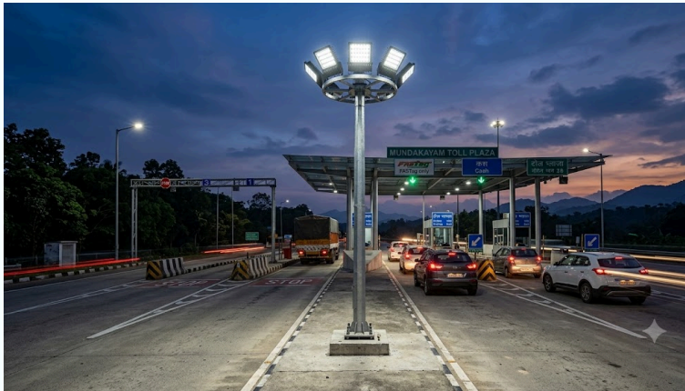
Toll Plaza Approach
